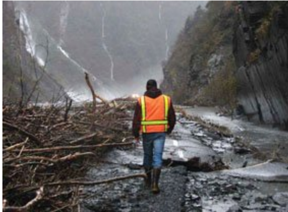
Flooding on the Alaska Richardson Highway
